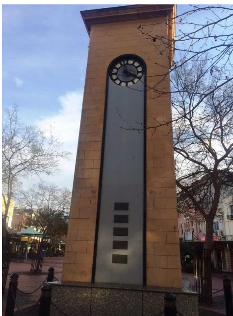
Campsie Clock Tower Memorial ( Photo from Monument Australia )
